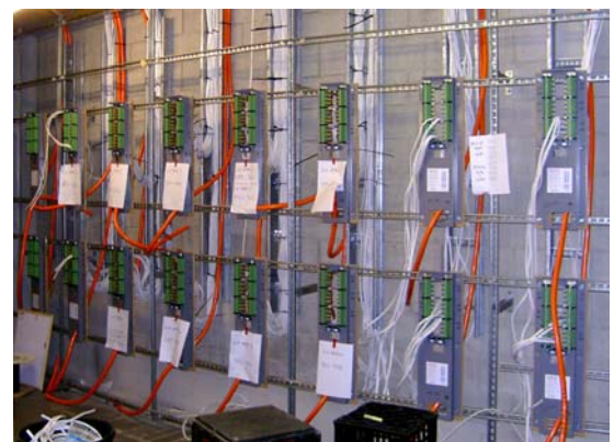
EKO Installation Frames during the wiring-in phase
